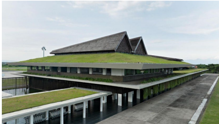
Gambar 1. 4 Banyuwangi International Airport Sumber. Archdaily (2022)
